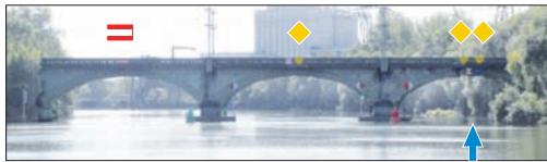
Pont rail SNCF
