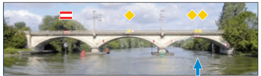
Pont rail SNCF
